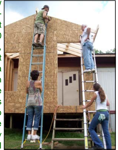
Construction at the Dalton home
