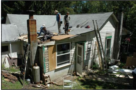
Construction at the McDaniel home in Philippi, WV
